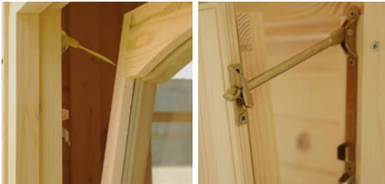
Windows open inwards and are provided with a tilt & turn system which can be opened using **TWO HANDS**.
