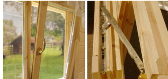
Windows open inwards and are provided with a tilt & turn system which can be opened using **ONE HAND**.
