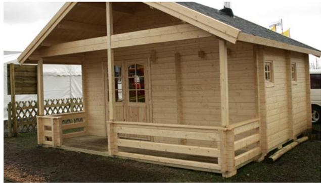
**BOUNDARIES (RAILINGS)** – made from the logs of the same size as used in walls (closed or open railings) or from strips.
