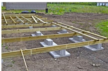
The foundation joists of the house are installed on the foundation. Later the walls are installed on the foundation joists. Usually the beams of the foundation joists are impregnated with a wood preservative. Impregnated foundation joists are not installed directly on the concrete but on bituminous material (not included in the delivery). This prevents penetration of moisture in wood.
